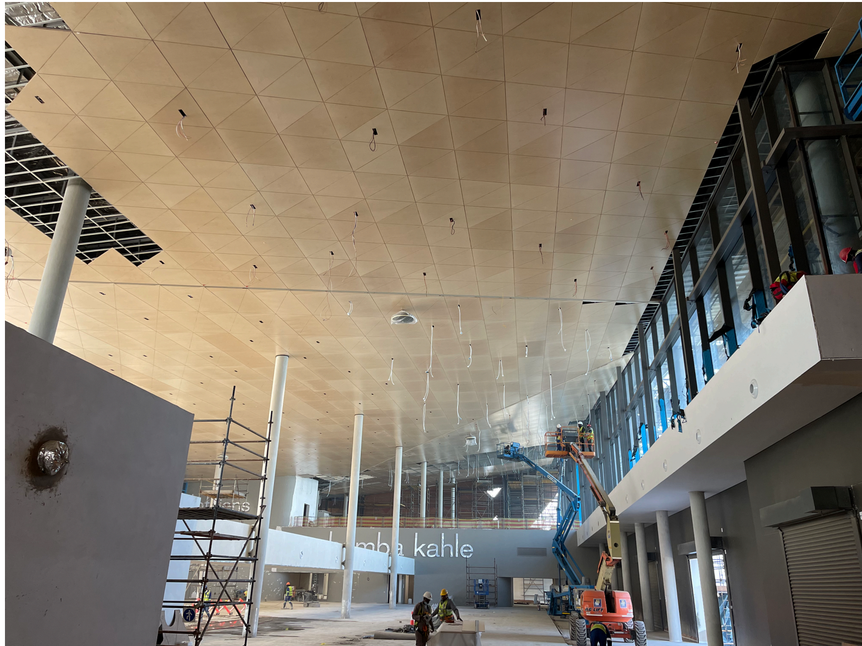
WIZA PLY CEILING CLADDING
