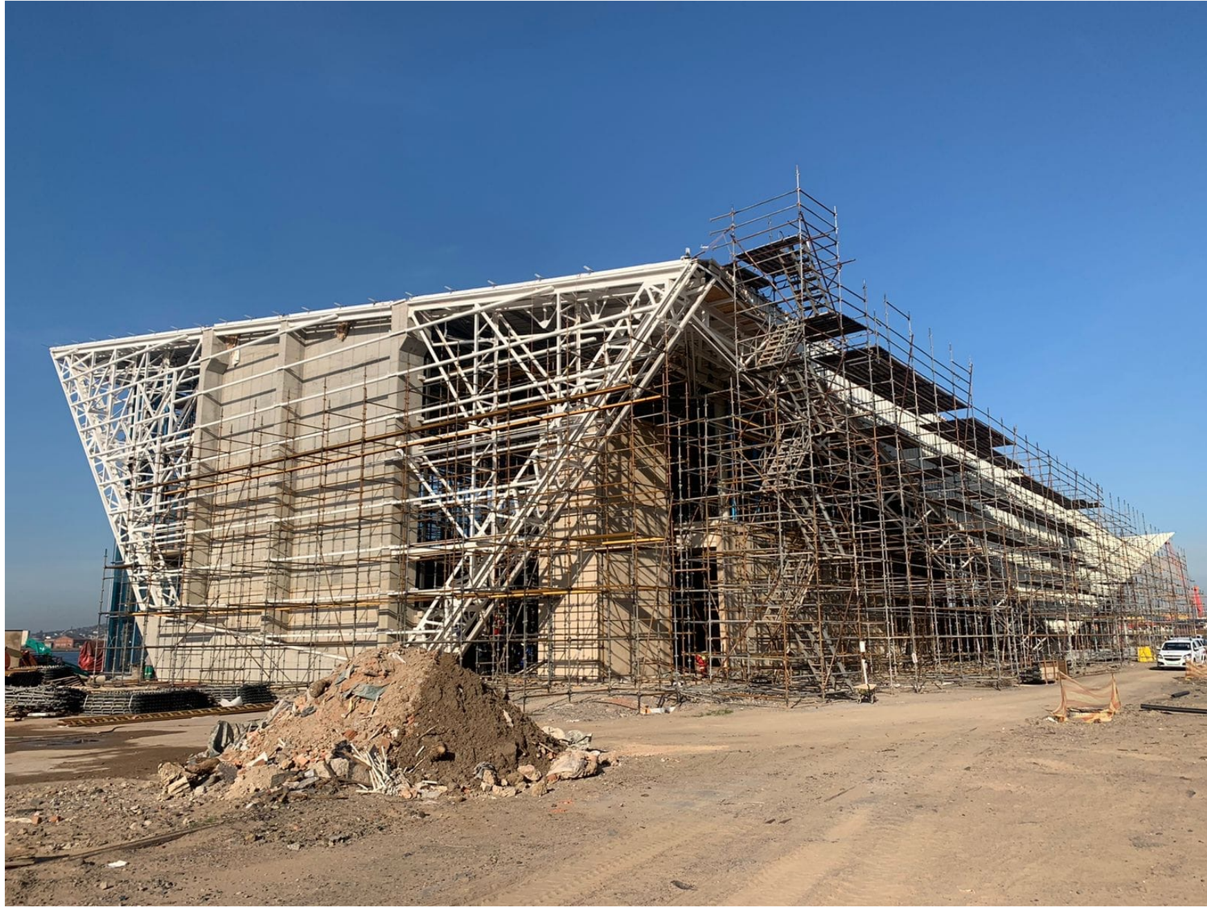
PRIMARY STEELWORK – SIDE WALL
