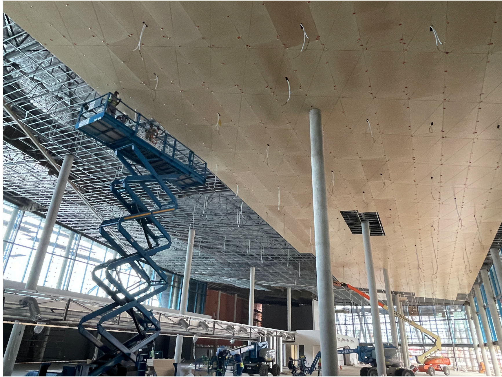
CEILING GRID AND WIZA INSTALLATION
