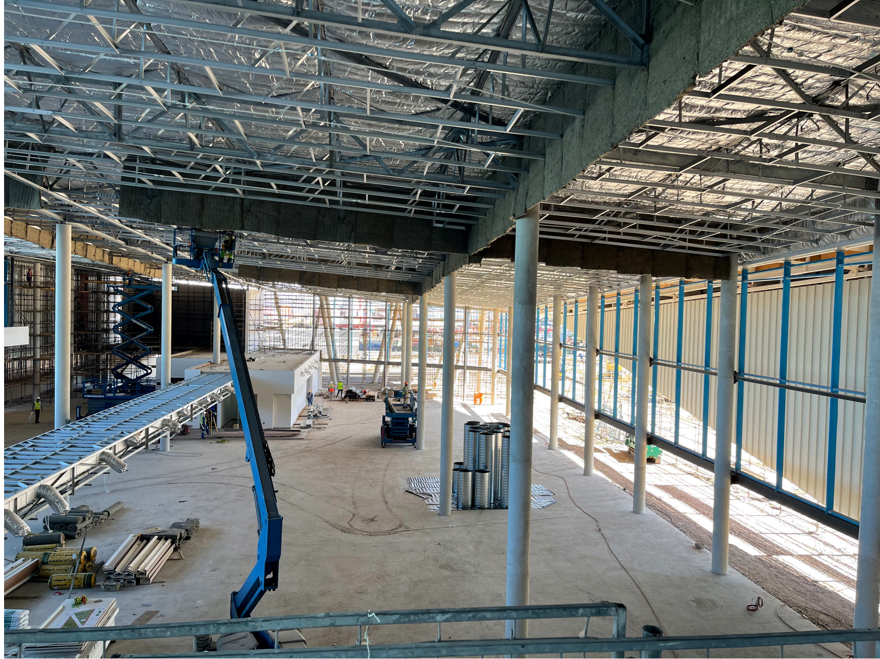
LSF,SUB GRID,LSF BULKHEAD
