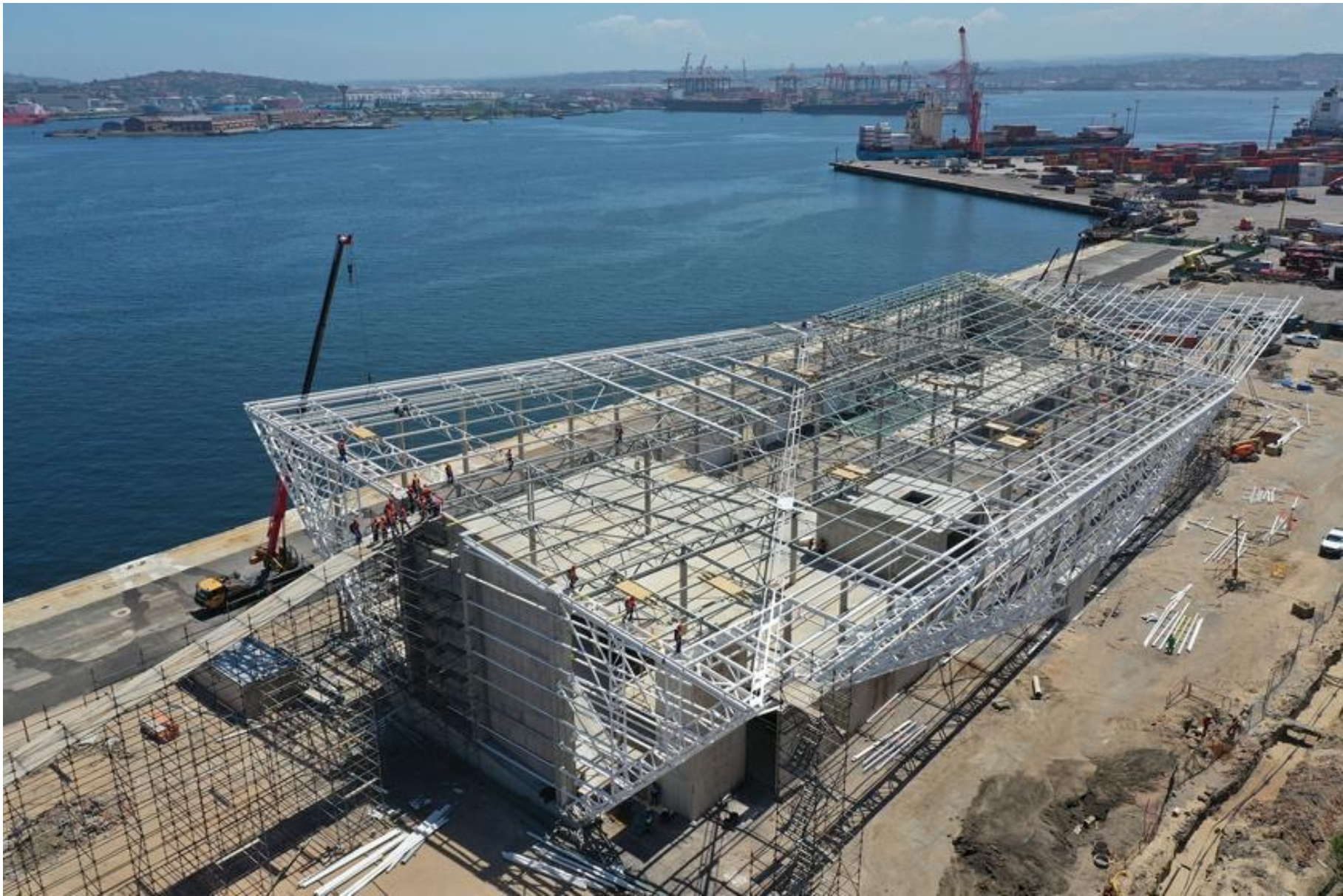
PRIMARY STEELWORK – MAIN BUILDING
