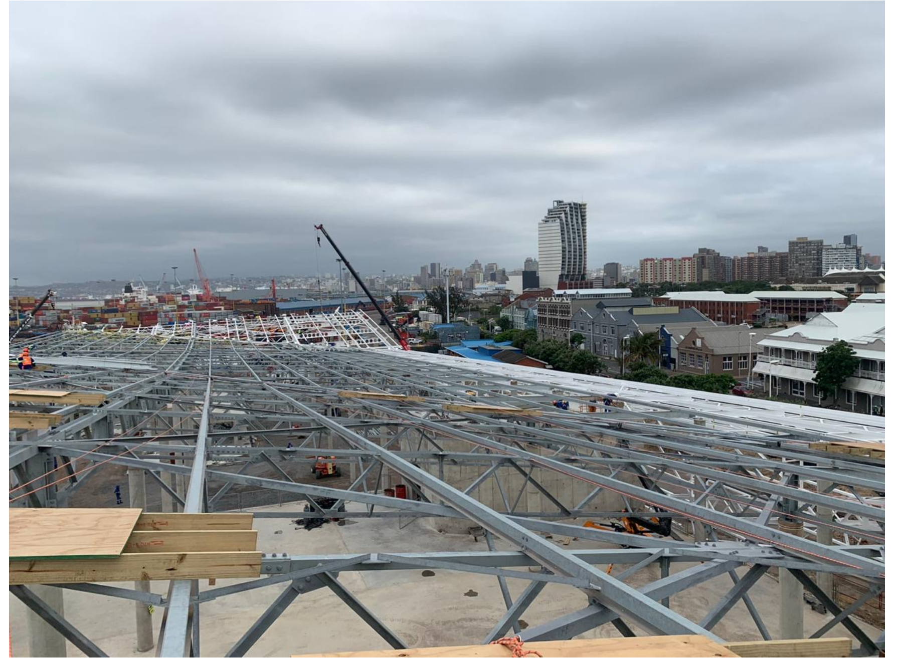
PRIMARY STEELWORK – ROOF STRUCTURE
