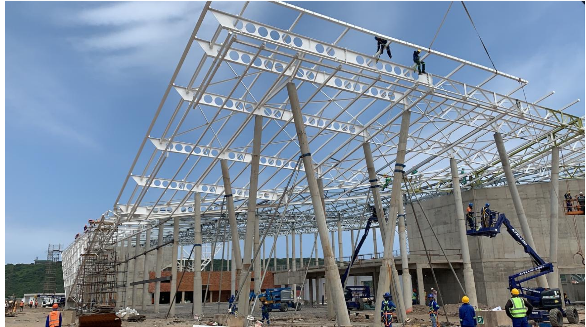
PRIMARY STEELWORK – ANGLED COLUMNS
