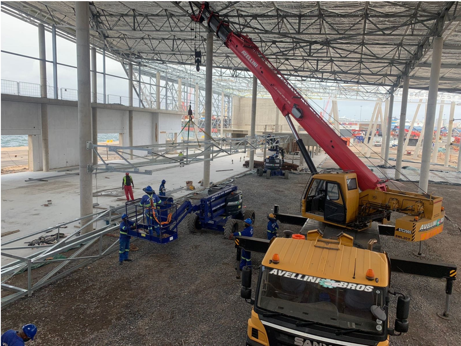
PRIMARY STEELWORK – INTERNAL SLIDING DOORS
