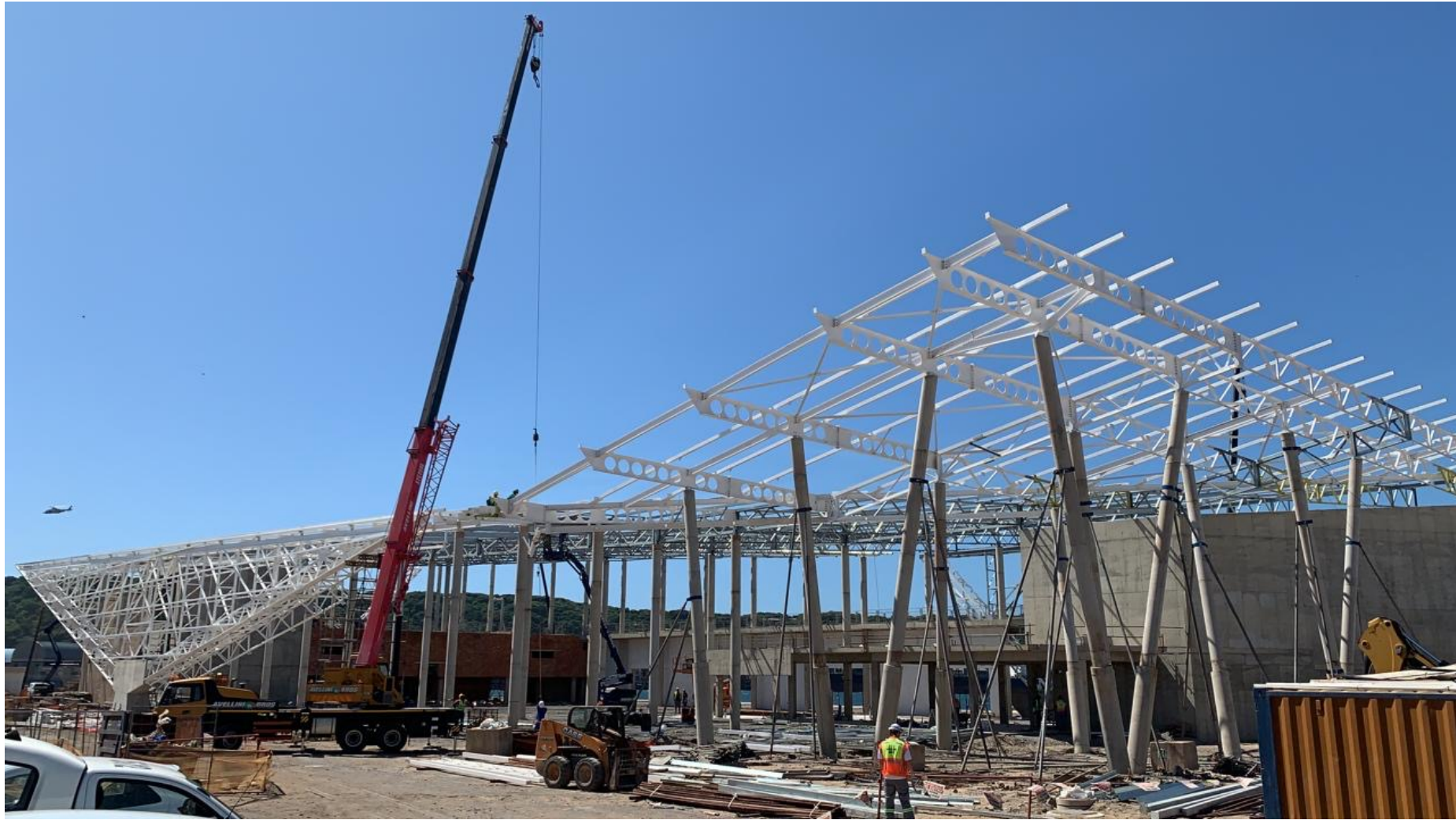
PRIMARY STEELWORK – ANGLED COLUMNS
